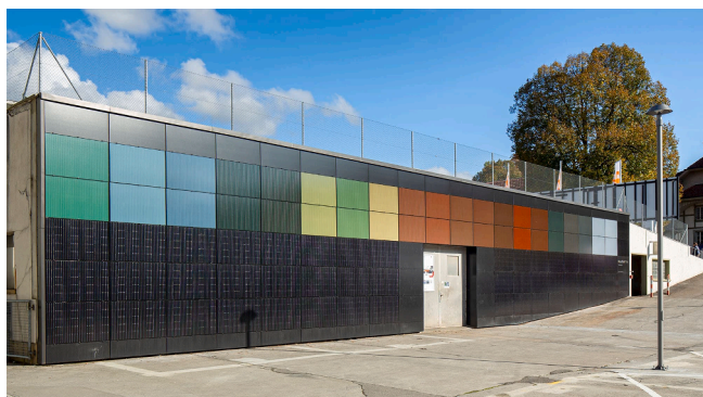
Fig. 2. Test installation of MegaSlate Flair DCP coloured modules in Bern with a varied range of colours. Image courtesy of 3S Swiss Solar Solutions AG [28].
